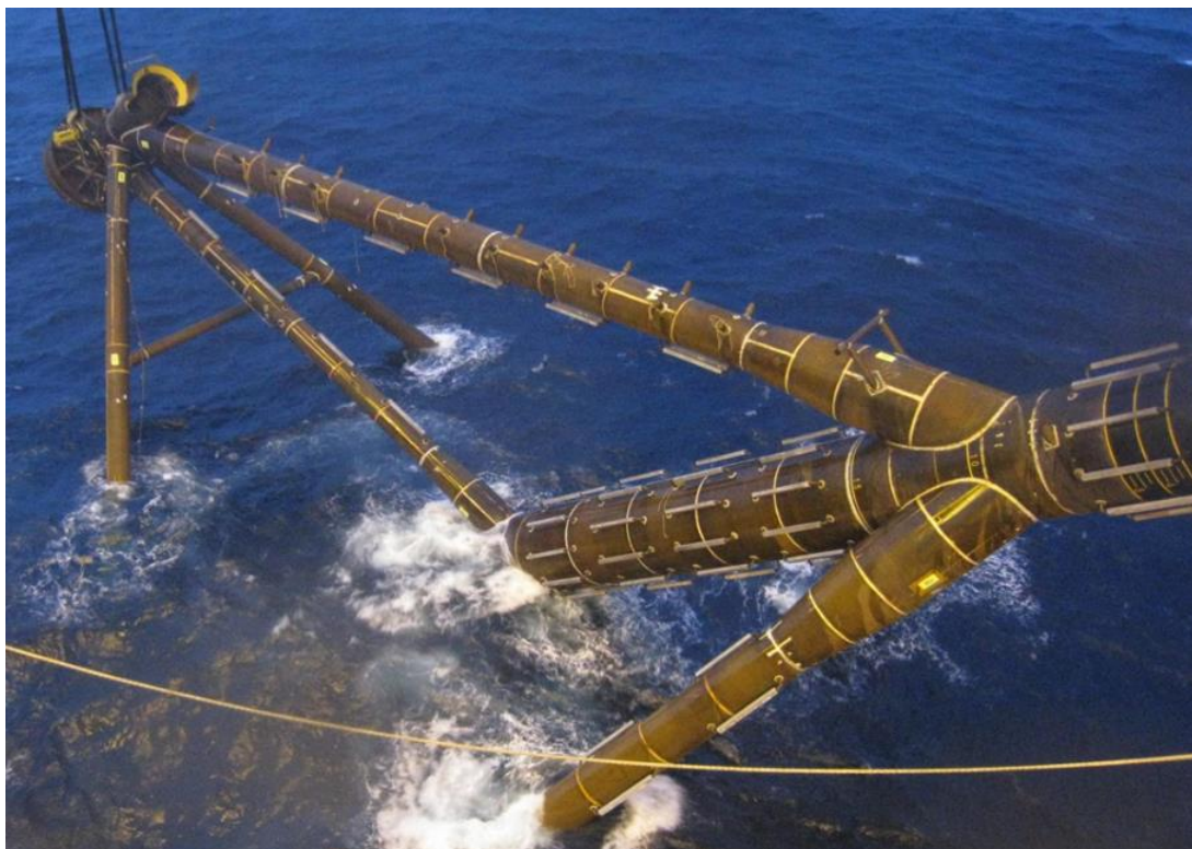
Figur 18-3 Jacket strukturen under installation.
